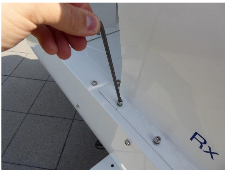
Use Allen key to fasten the air baffles.
