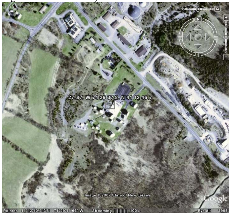
Figure 10. Aerial View, site #5
