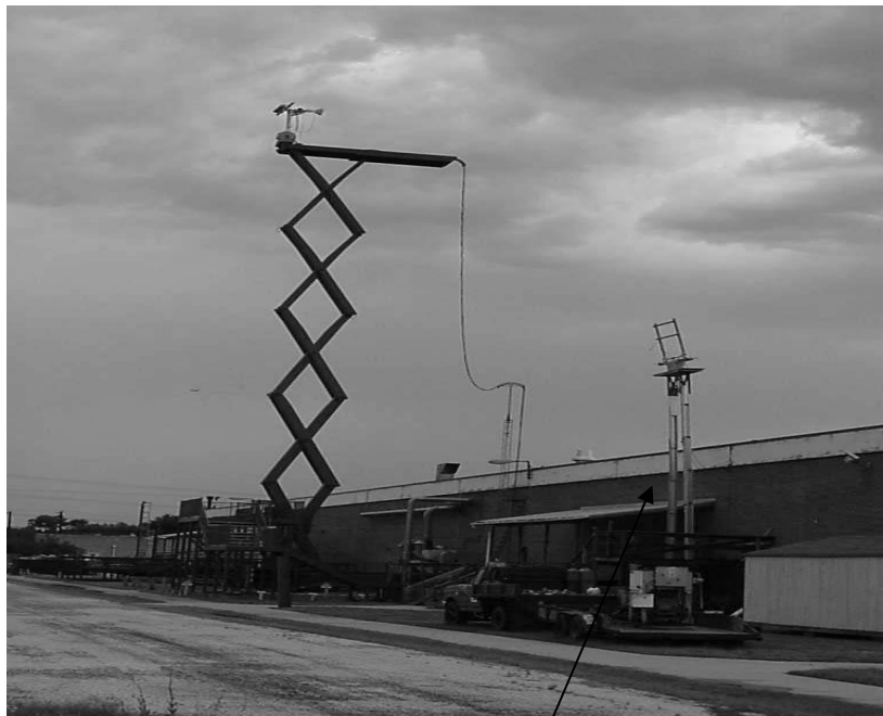
Site 2 Antenna On the Right
